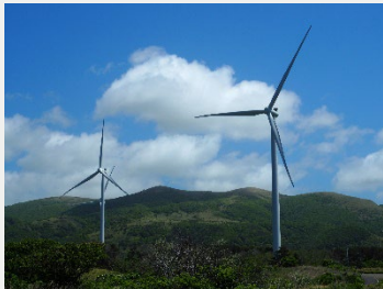
ReENE Matsumae Wind Power Plant (Hokkaido) Rated capacity: 41MW (Operation started in FY2019)
