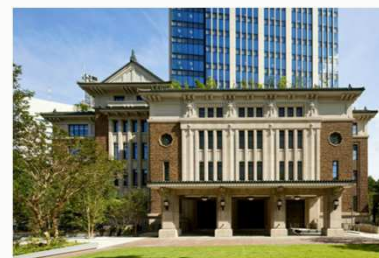
Exterior of Kudan-Kaikan Terrace (preserved area)
