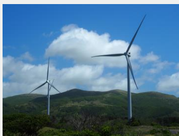
ReENE Matsumae Wind Power Plant (Hokkaido) Rated capacity: 41MW (Operation started in FY2019)
