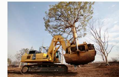
Transplanting work using a TPM machine
