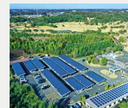
ReENE Shibayama Golf Club Solar Power Plant
