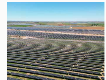
Manzanares solar power plant (Ciudad Real, Spain)
