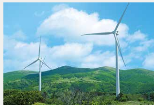
ReENE Matsumae Wind Power Plant
