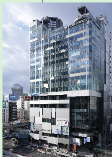
Shibuya Fukuras Shibuya-ku Office/Commercial Total floor space: 59 Completion in December 2019
