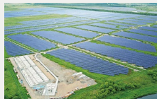
ReENE (Solar power generation facilities)
