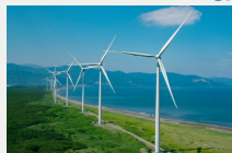
ReENE (Wind power generation facilities)
