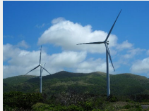
ReENE Matsumae Wind Power Plant (Hokkaido) Rating capacity: 41 MW (Operation began in FY2019)
