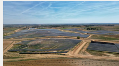
Valdecarretas Solar Power Plant (Spain) Rated capacity: 38 MW (Commercial operation started in December 2023)
