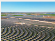
Manzanares Solar Power Plant (Spain) Rated capacity: 40 MW (Commercial operation started in June 2023)
