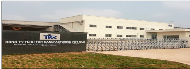
Exterior view of TKR Vietnam
