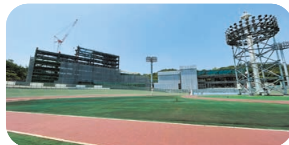
Construction site of the Tamano Velodrome
