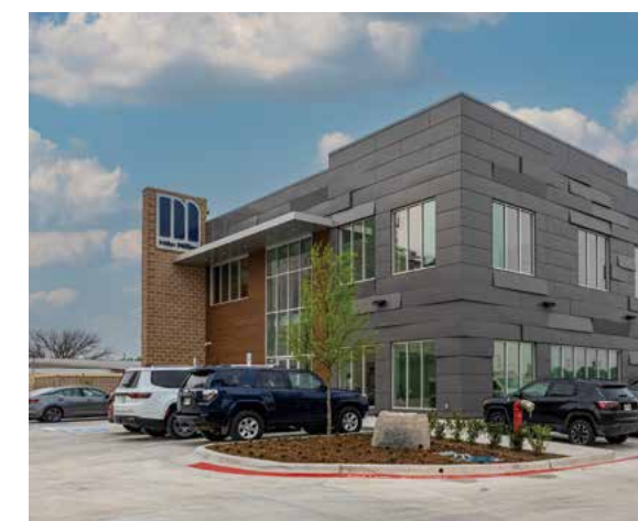
Innovation & Technical Center (ITC)
