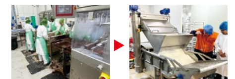
Automation equipment has been installed for various processes
