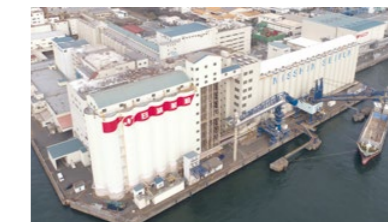
The Nisshin Flour Milling, Tsurumi Plant
