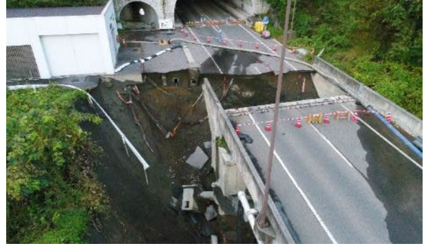
Disaster recovery of Gonbee-Toge Pass
