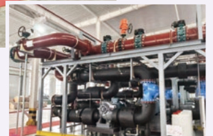
Example of prefabricated module installation
