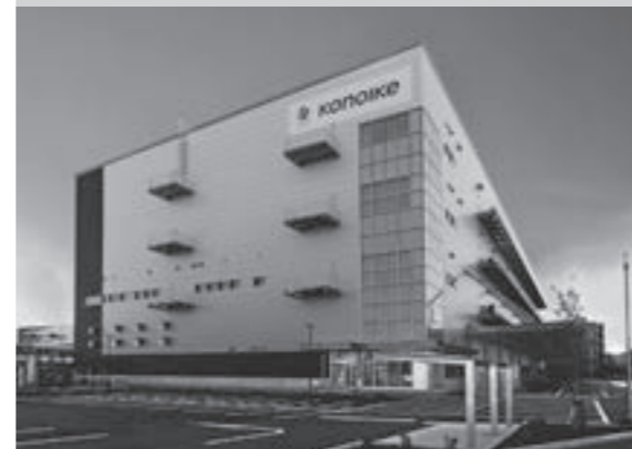
Konoike Transport Co., Ltd. TechnoLogis Makuhari Office Chiba Prefecture
