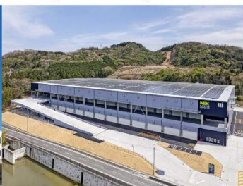
UI Konan Logistics Center Phase 1
