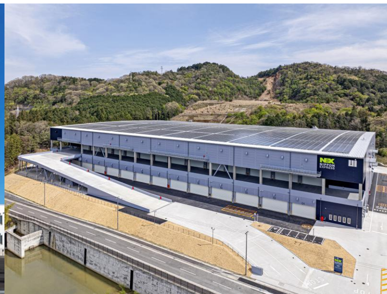
UI Konan Logistics Center Phase 1
