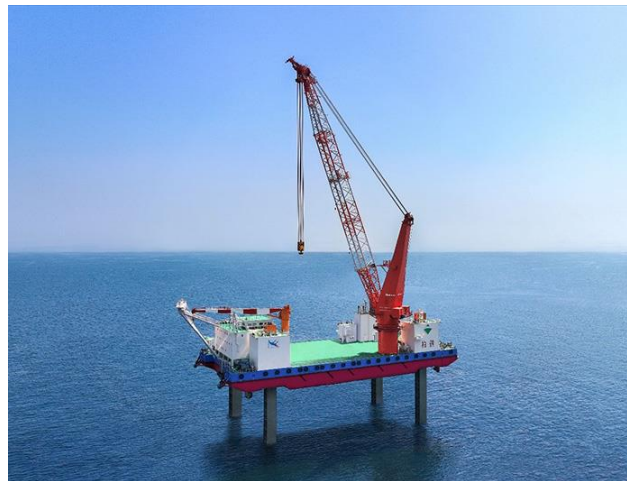
Completed SEP vessel “Hakkaku”
