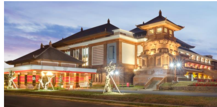
Construction of the Bali Theater
