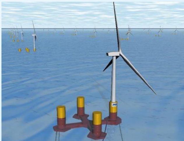
Semi-submersible floating structure (Courtesy of the Japan Marine United Corporation)
