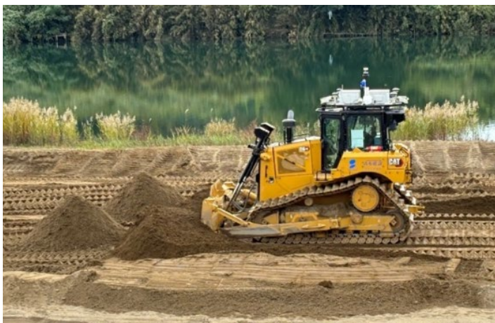
Demonstration Project (Leveling a Pile of Soil and Sand)
