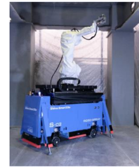
Semi-dry fireproof coating spray robot, Robo-Spray II
