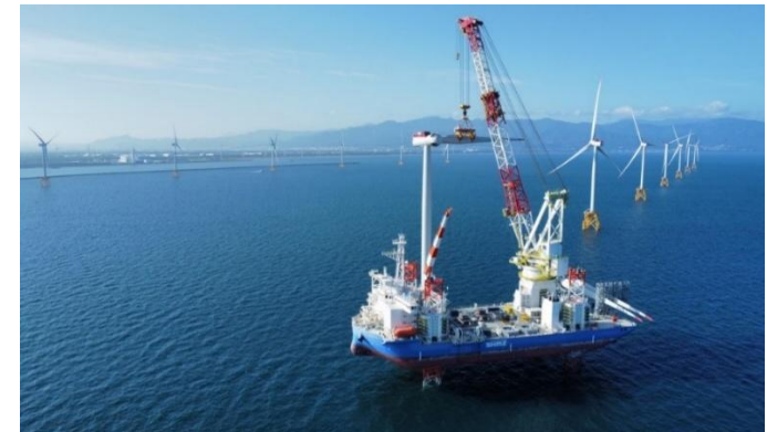
Hai Long 2 Offshore wind farm construction project (Taiwan)
