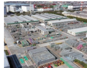
Head Office equipment and materials center (Funabashi City, Chiba Prefecture)
