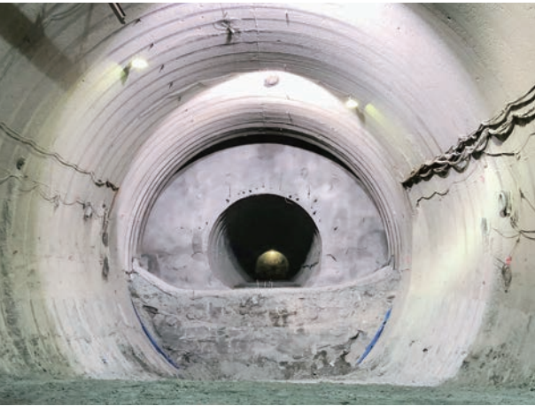
Cross-section closure of main tunnel in center drift advancing method Otonaka tunnel excavation work in Otoineppu Village on National Route 40 (Otoineppu Village to Nakagawa Town in Nakagawa District, Hokkaido)
