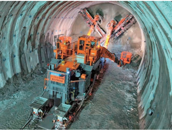
Fully mechanized rock bolt work (using "Rock Bolter") Maki Tunnel work on Tokai Hokuriku Expressway (Nanto City, Toyama)
