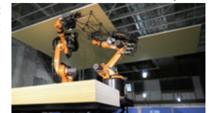
Robo-Buddy installing a ceiling
