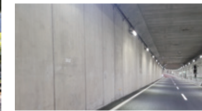
Labor/saving for construction of the "Large Section Box Calvert" by the "Hybrid Half Pre-casting Method": At the A-ramps for turn off of Keiyo Junction in Tokyo-Gaikan Expressway
