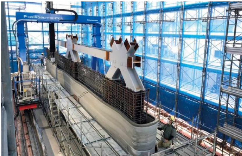
On-site 3D printing construction
