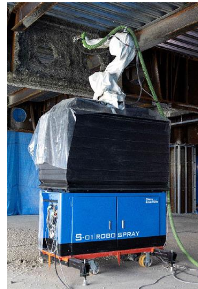
Semi-Dry Fireproof Covering Spraying Robot "Robo-Spray"
