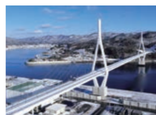
Kesenuma Bay Crossing Bridge (Kesenuma City, Miyagi)
