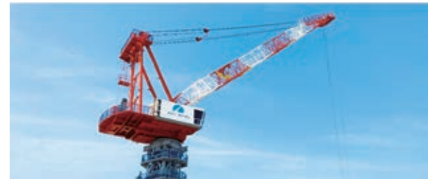
Mainstay large tower crane
