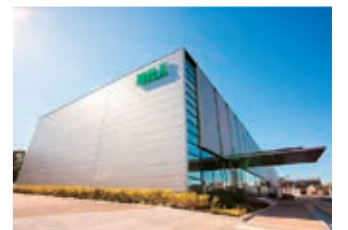
Head Office equipment and materials center (Funabashi City, Chiba Prefecture)
