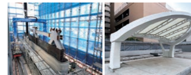
On-site 3D printing construction
