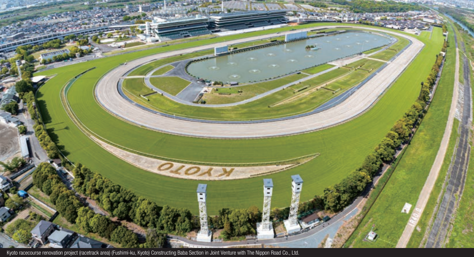
Kyoto racecourse renovation project (racetrack area) (Fushimi-ku, Kyoto) Constructing Baba Section in Joint Venture with The Nippon Road Co., Ltd.
