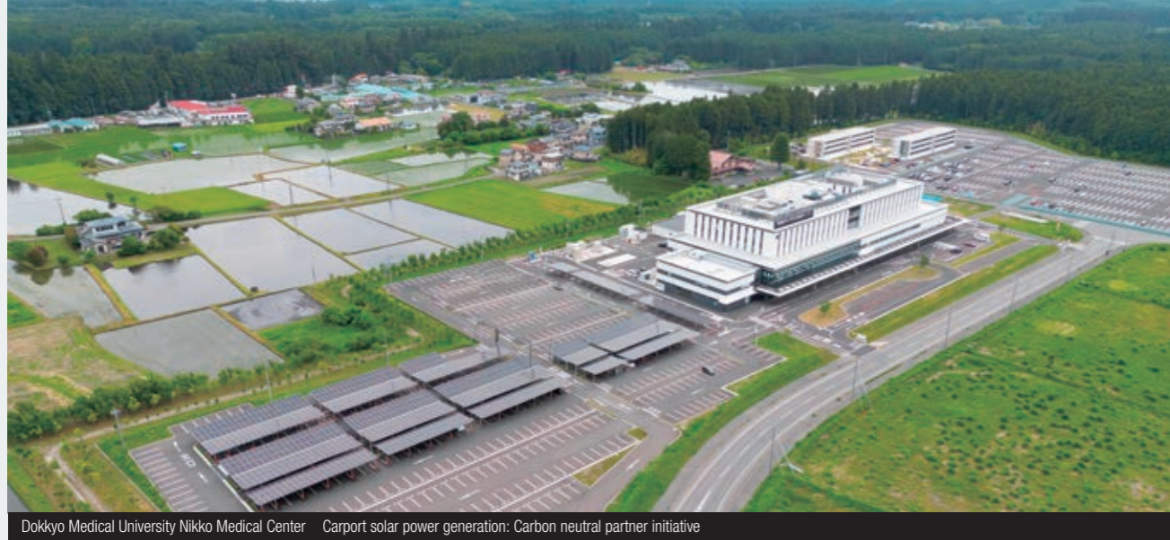
Dokkyo Medical University Nikko Medical Center Carport solar power generation: Carbon neutral partner initiative
