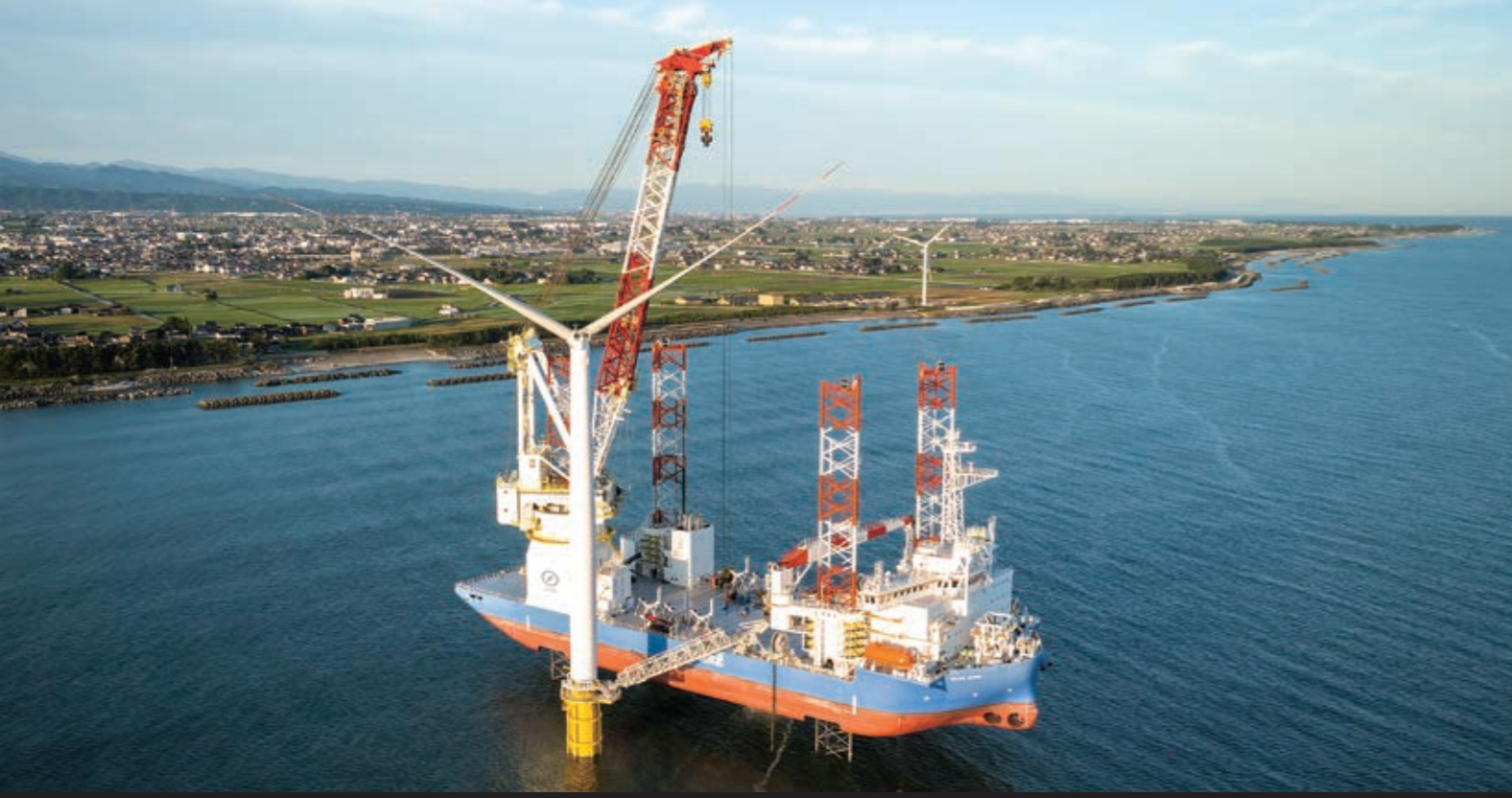
SEP vessel BLUE WIND for construction of offshore wind farms
