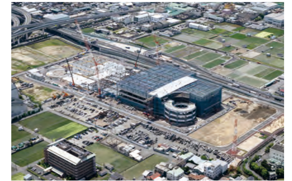
S-LOGI Matsubara Construction Site (Matsubara City, Osaka Prefecture)
