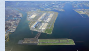
2010 Tokyo International Airport D-runway Large-scale offshore runway featuring hybrid structure of reclaimed land and pier, uncommon around the world (photo courtesy of Haneda re-expansion D runway JV)
