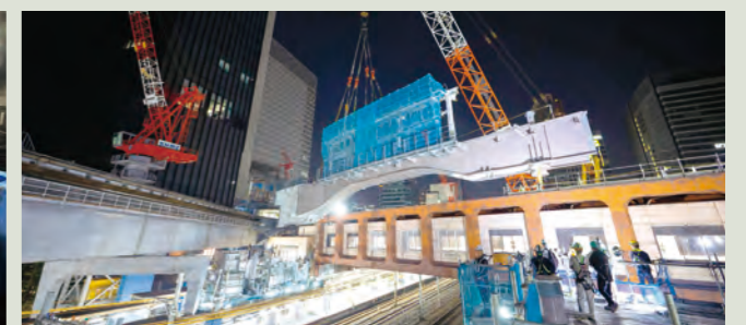
Walkway girder installation above the rail lines
