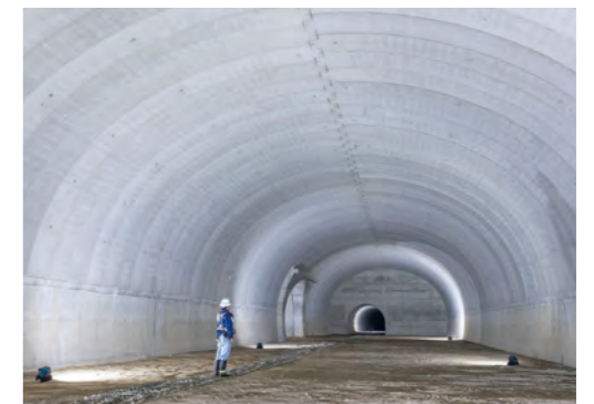
One of the largest precast linings in Japan (intermediate pump room) (Aso City, Kumamoto Prefecture)
