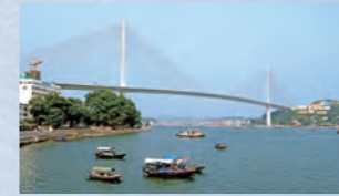
2006 Bai Chay Bridge (Vietnam) A giant 903-meter cable-stayed bridge over Ha Long Bay, a World Natural Heritage site. Various wind protection measures were implemented to address the challenges of regions prone to frequent typhoons.
