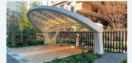
Parking lot roof structure (Smart Innovation Ecosystem NOVARE)
