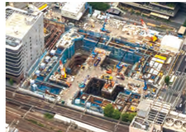
Demonstration underway at the Torch Tower work site under the Tokyo Metropolitan Government's subsidy program to promote commercialization of biofuel use
