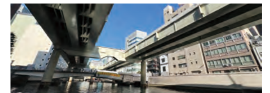
Completion of bridge beam and bridge pier removal
