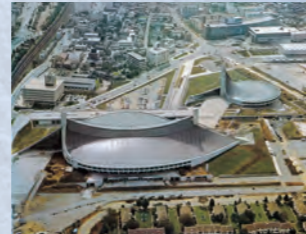
1964 National Indoor General Stadium Main Gymnasium Achieved a column-free space with an unprecedented wire-suspended roof structure.
