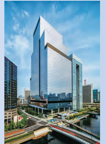
2025 BLUE FRONT SHIBAURA (TOWER S) The first tower of the twin towers with a view of the Tokyo Bay area. The first application of our proprietary vibration control technology, BILMUS.
