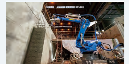
Construction at Nippon Steel Corporation's Setouchi Works, Hanshin Area (Sakai)
