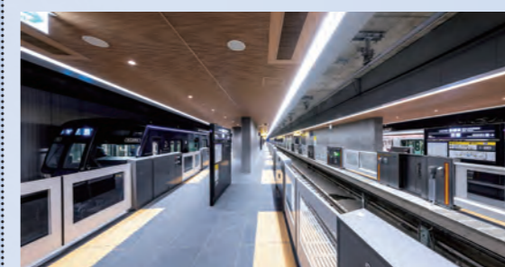
2024 Sotetsu/Tokyu Shin-yokohama line, Shin-Yokohama Station, etc. Making full use of digital tools, we have improved productivity and achieved more efficient and advanced construction management.
