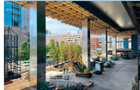
View of the 18-meter span external columns on the first floor
