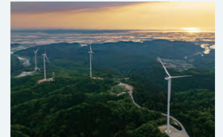
The first application at Nakasato Wind Project (photo provided by Studio Quaria)
