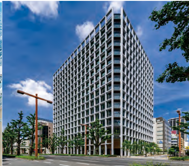
Nagoya Shimizu Fukoku Seimei Building (Nagoya City, Aichi Prefecture)
