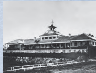
1868 Tsukiji Hotel Japan's first authentic Western-style hotel. In addition to its financing and construction, the company managed the hotel after its completion.
