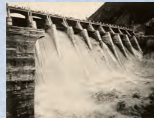
1936 Yahagi Suiryoku Yasuoka Hydroelectric Power Station Our first challenge in undertaking a full-scale dam construction project. It turned into a battle against the forces of nature.
