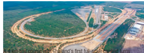
4 km test course with Thailand's first full-scale banked turns
