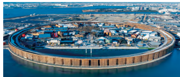
Introduction of 100% pure biofuel in the construction work for the Expo 2025 Osaka, Kansai, Japan (utilizing subsidies from Osaka Prefecture)
