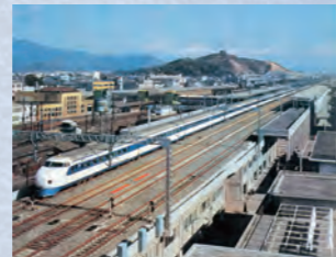
1964 Tokaido Shinkansen Shizuoka Station Elevated Bridge Participation in a national transportation infrastructure development project to connect East and West Japan
