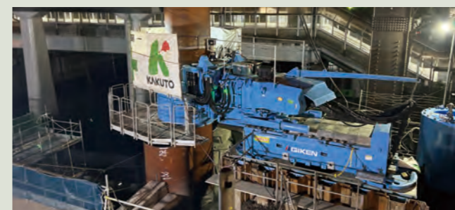
Gyropress use in revetment reconstruction
