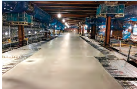
Preconstructed floor for basement materials transportation
