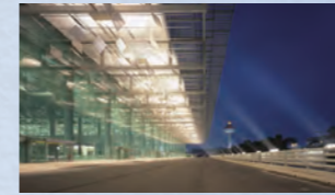
2007 Changi Airport Terminal 3 (Singapore) A terminal in a key economic hub of Southeast Asia. The method of lifting up steel frame trusses measuring 300 meters wide and 215 meters deep, was a first in the world
