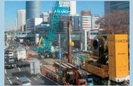
Steel-reinforced continuous underground wall components installed along Circular Line 2
