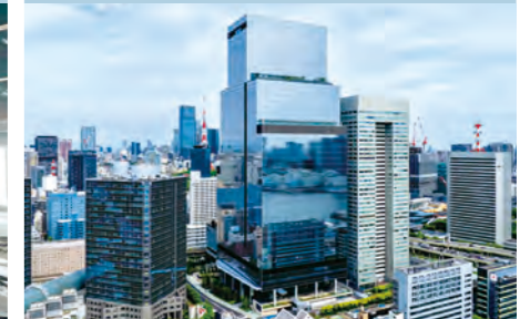
External view of completed building
