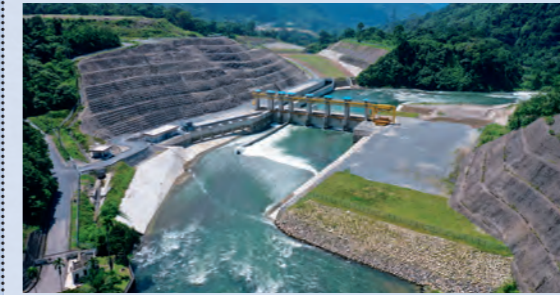
2024 Asahan No.3 Hydroelectric Power Plant (Indonesia) A multi-disciplinary project involving a 10.9 km tunnel, an underground power station, and shaft construction. Actively leveraging ICT technologies, including BIM models.
