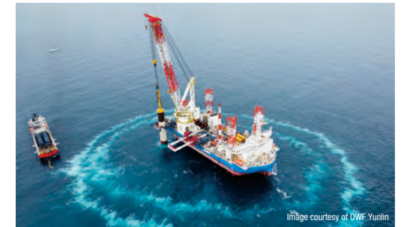
Bubble curtain of Yunlin Offshore Wind Farm construction project (chartered) (Taiwan)
