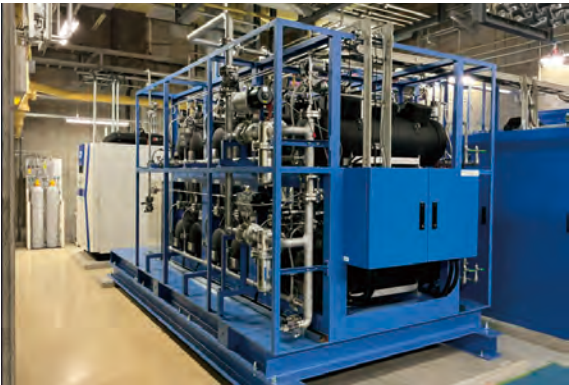
Hydro Q-BiC hydrogen storage alloy tank (inside the Aomi Minami Plant of Tokyo Rinkai Heat Supply Corporation, Tokyo)
