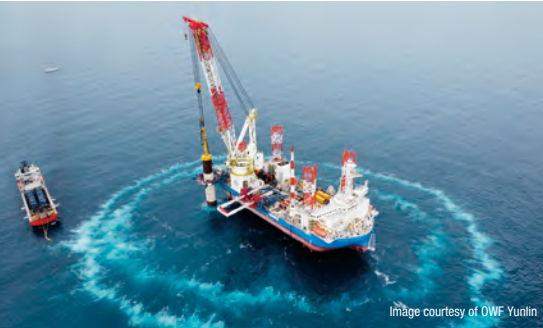
Bubble curtain of Yunlin Offshore Wind Farm construction project (chartered) (Taiwan)
