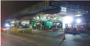
Multi-axle transporter installation between P1 and P2 of Ohibashi-Nishi Viaduct (commissioned by the Chugoku Regional Development Bureau, Ministry of Land, Infrastructure, Transport and Tourism)
