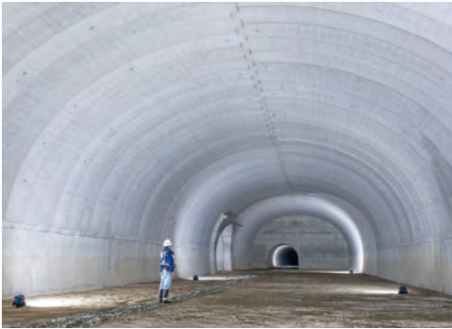
One of the largest precast linings in Japan (intermediate pump room) (Aso City, Kumamoto Prefecture)
