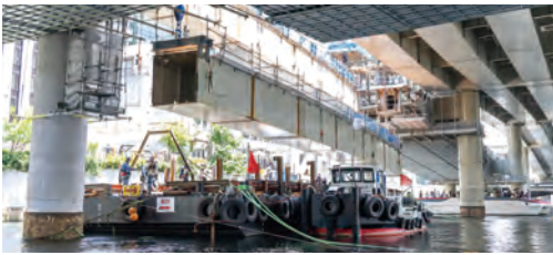
Removing a steel bridge beam by suspending and lowering it with the use of a barge (Chuo Ward, Tokyo)
