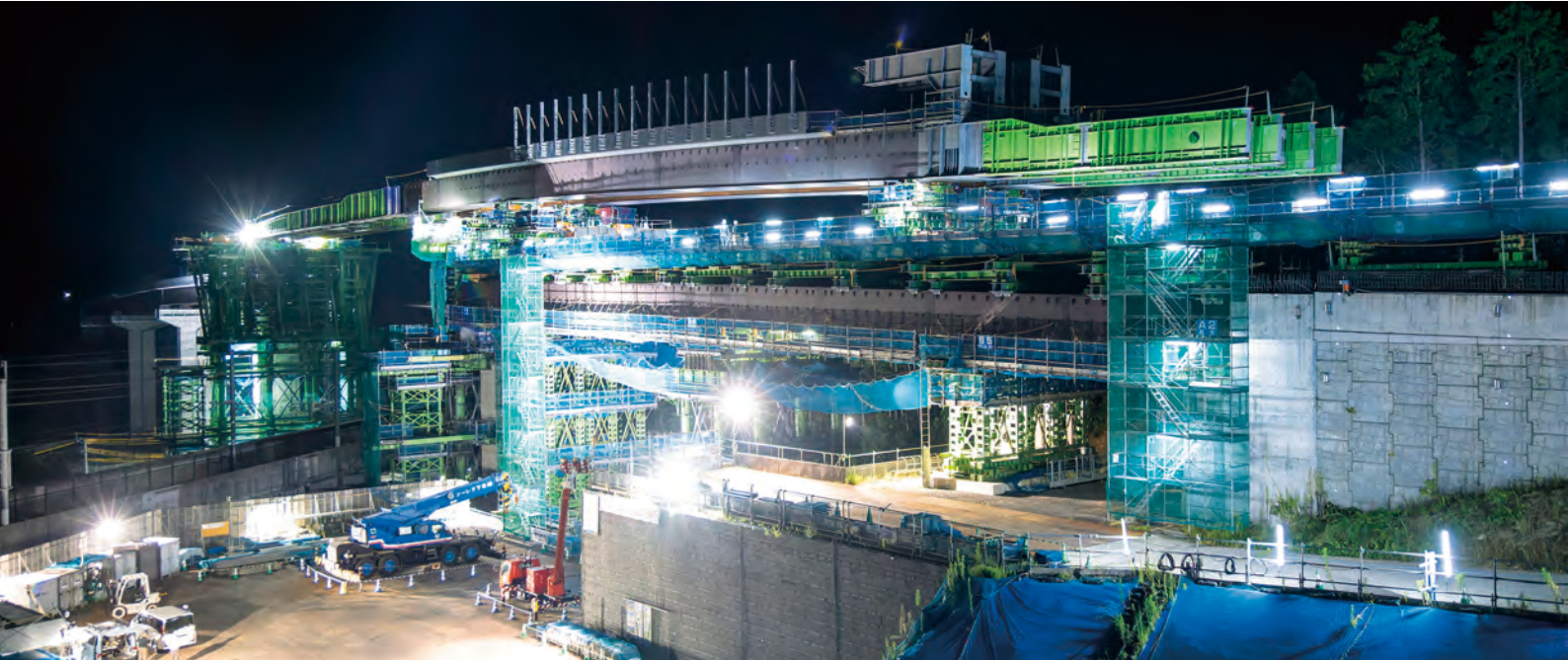
Construction of the Kojo overbridge No. 2 in the Shin-minamata Station precincts and three other works (Minamata City, Kumamoto Prefecture), with bridge erection across the Kyushu Shinkansen using the launching erection method
