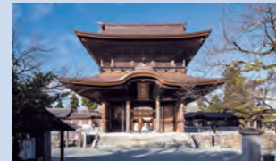
2023 Preservation and Repair Work on Ronon Gate of Aso Shrine Rebuilt the gate, which was completely destroyed in the 2016 Kumamoto earthquake. The materials were repaired wherever possible and reused.
