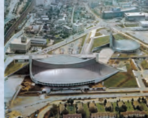
1964 National Indoor General Stadium Main Gymnasium Achieved a column-free space with an unprecedented wire-suspended roof structure.
