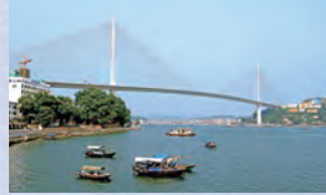
2006 Bai Chay Bridge (Vietnam) A giant 903-meter cable-stayed bridge over Ha Long Bay, a World Natural Heritage site. Various wind protection measures were implemented to address the challenges of regions prone to frequent typhoons.
