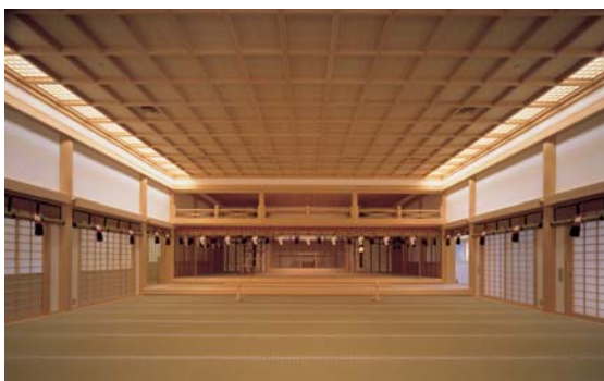
The interior of Ise Jingu Geku Kaguraden (Hall for special prayer) built by the sawmill. Although steel was used for the structural framework to increase durability, our craftsmen fashioned the cedar wood around the framework to give the appearance of an all-wood structure.
