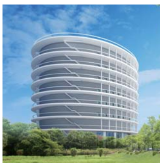
The balconies around the exterior increase the strength and resistance of the structure as well as protecting the building from colliding flotsam.
