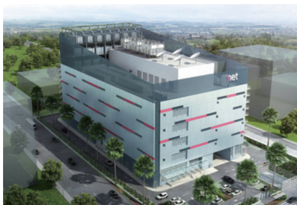
Woodlands Data Center, Singapore
