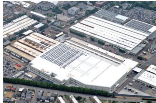
Located on a 710,000m 2 site, the Awazu Plant is one of the largest factories in Japan. The new assembly plant is the large building in front with solar panels on the roof.
