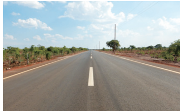
The Project for Improvement of the Living Environment in Southern Area of Lusaka
