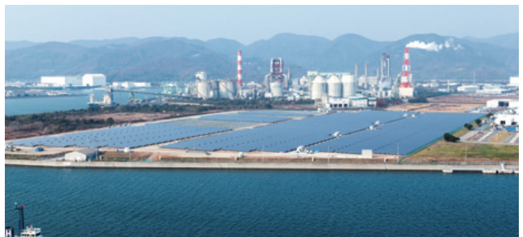
The Ako Mega-solar Power Plant in Hyogo prefecture
