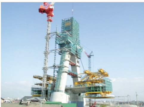
A main pylon under construction
