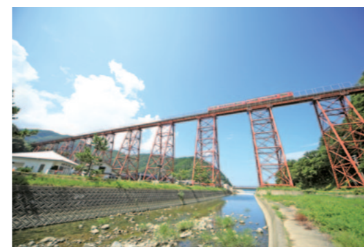
The old viaduct before replacement. The slender, linear design of the new viaduct evokes the look of the old structure.
