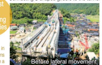
Connecting S-shaped girders to the tunnel
