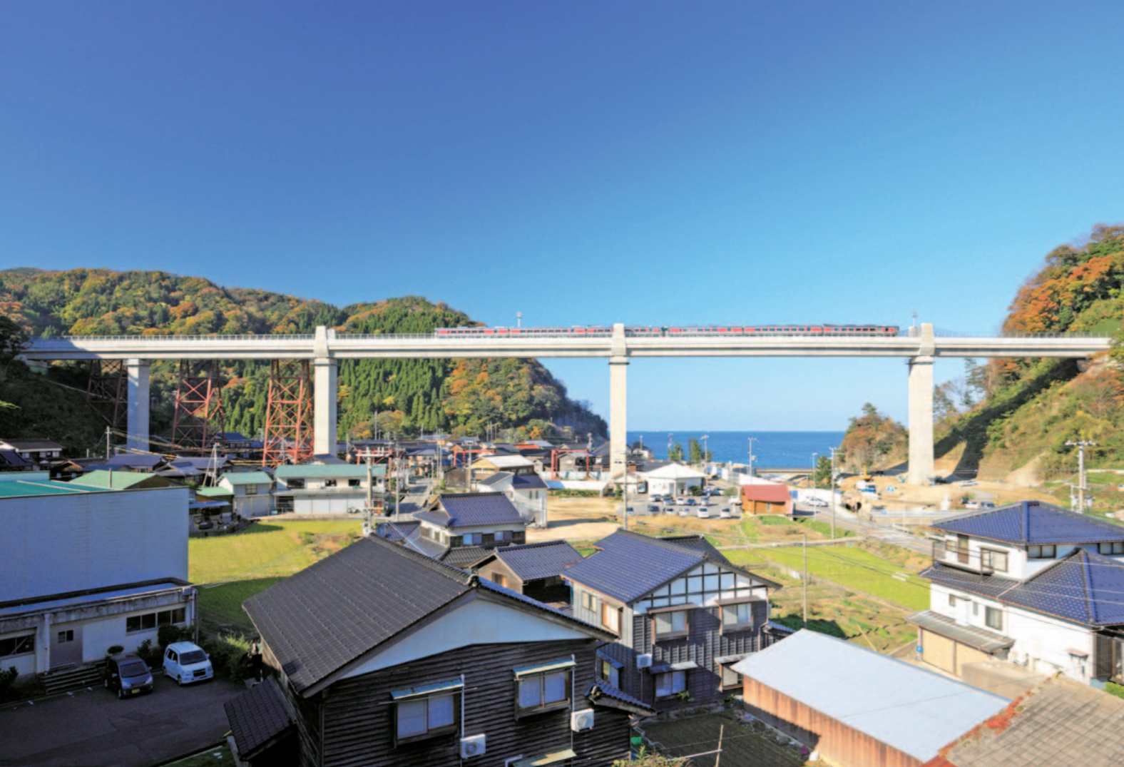
A new viaduct with 15-millimeter windbreak walls on both sides so that trains can pass, even at wind speeds of 30 meters/second. Acrylic sheets preserve passenger views from passing trains.
