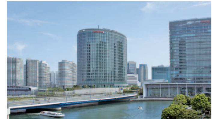
The building as seen from Bay Quarter Yokohama, at the East Exit of JR Yokohama Station
