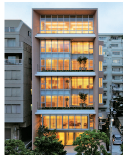
The exterior of the clinic. The two pairs of floors—the third and fourth floors and the fifth and sixth floors—are designed to resemble two two-story homes stacked on top of each other.
