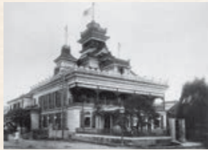
1872 Dai-ichi National Bank Japan's first bank building construction
