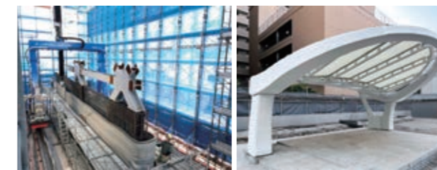
On-site 3D printing construction
