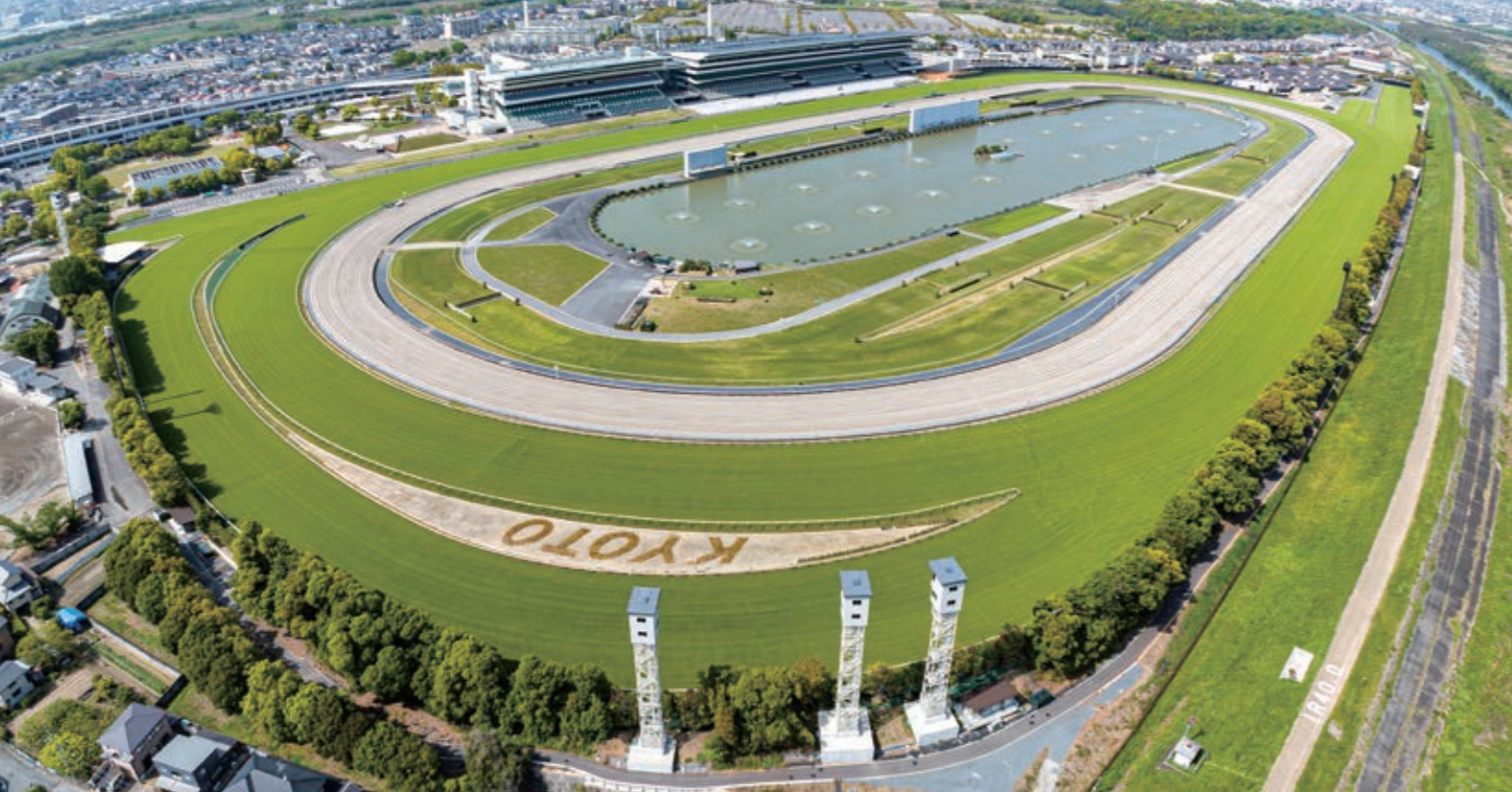
Kyoto racecourse renovation project (racetrack area) (Fushimi-ku, Kyoto) Constructing Baba Section in Joint Venture with The Nippon Road Co., Ltd.
