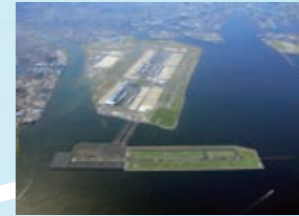
2010 Tokyo International Airport D-runway Large-scale offshore runway featuring hybrid structure of reclaimed land and pier, uncommon around the world (photo courtesy of Haneda reexpansion D runway JV)
