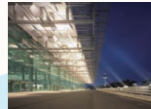
2007 Changi Airport Terminal 3 (Singapore) The method of lifting up steel frame trusses measuring 300 meters wide and 215 m deep, was a first in the world
