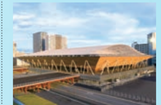
2019 Ariake Gymnastics Centre One of the world's largest timber-framed roofs. Designed to communicate the Japanese culture of using wood and sustainability.
