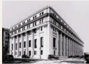
1920 Mitsui Main Building Beginning of full-scale mechanized construction (photo courtesy of Mitsui Bunko Public Interest Incorporated foundation)
