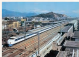
1964 Elevated Bridge at Shizuoka Station on Tokaido Shinkansen Line Participation in a major national project to connect East and West Japan
