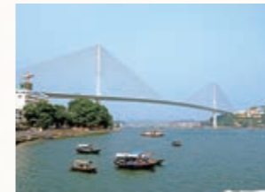
2006 Bai Chay Bridge (Vietnam) A giant 903-meter cable-stayed bridge over a World Heritage Site
