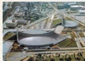
1964 Main Gymnasium of the National Indoor General Stadium Unprecedented suspension roof structure
