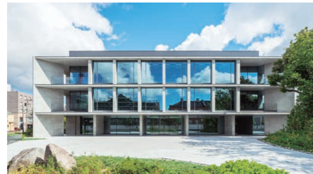
Exterior view of the Shimizu Hokuriku Branch Office Building
