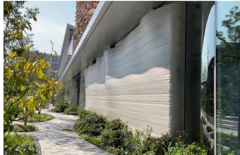
Easy to create free-form curved surfaces, which was difficult with conventional construction methods.
