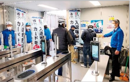
Activities at the entrance gate of a construction site
