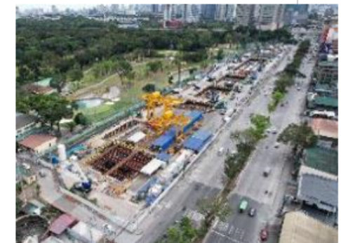
Manila Metro Project (The Philippines)
