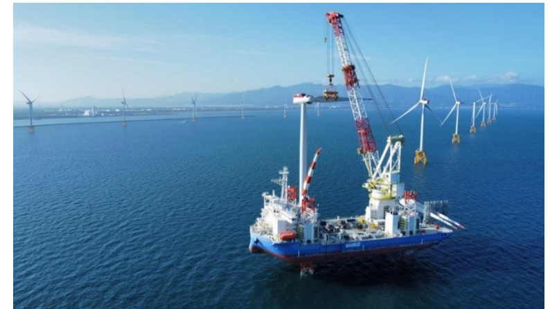
Ishikari Bay New Port Offshore Wind Farm Constructed by our self-propelled SEP vessel "BLUE WIND"
