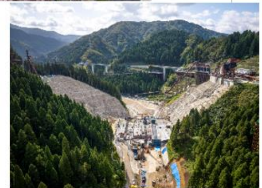
Asuwagawa Dam, Fukui Pref.
