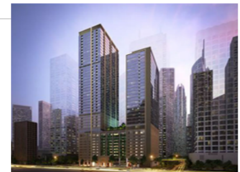
Branz Mega Kuningan Project (Indonesia)
