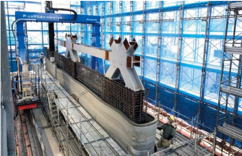
On-site 3D printing construction
