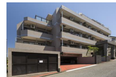
Hachioji-shi Income-generating Apartment
