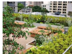
Toranomon Tosei Building (Build in 2006 as a office)
