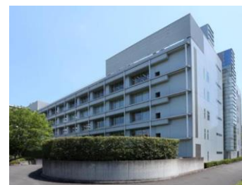
Itabashi-ku Income-generating Building
