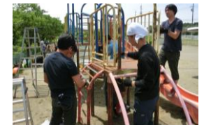
Painting rusted playground equipment at nursery center
