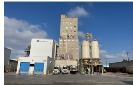
The Los Angeles Plant of Miller Milling Company
