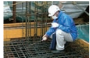
Inspection by a technical staff member
