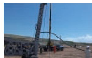
The methane gas recovery facility under construction in Armenia
